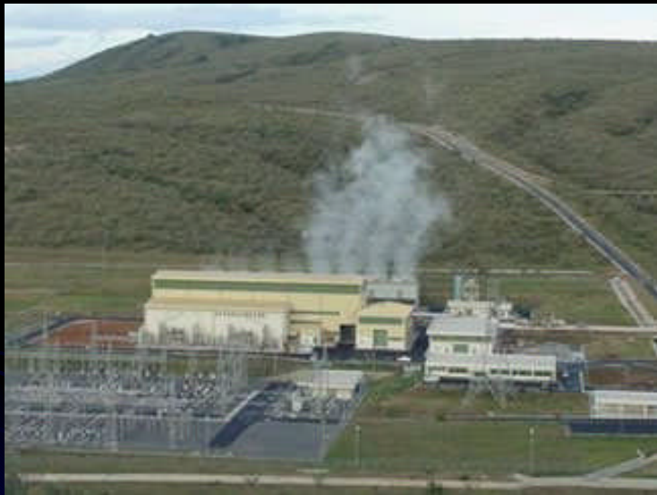
A geothermal plant in Kenya.
