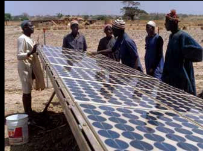
A photovoltaic power system near the Volta River.
