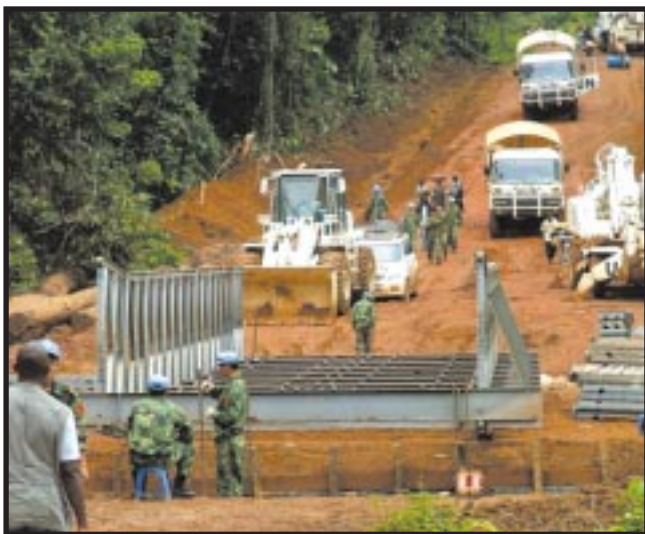
Acrow Bridge being assembled by UN forces in Liberia, 2005.
